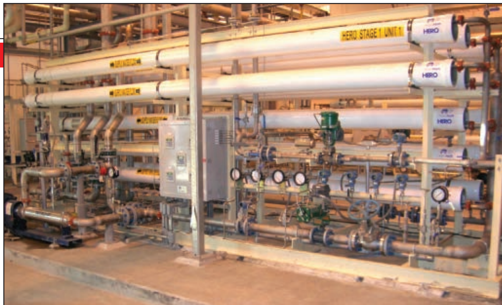
FIGURE 2. Aquatech's HERO system is a reverse osmosis technology designed to purify difficult-to-treat feed waters. In a HERO system, RO membranes are operated in a high pH environment and hence, in a continuous cleaning mode, eliminating the potential foulants and resulting in improved overall performance
